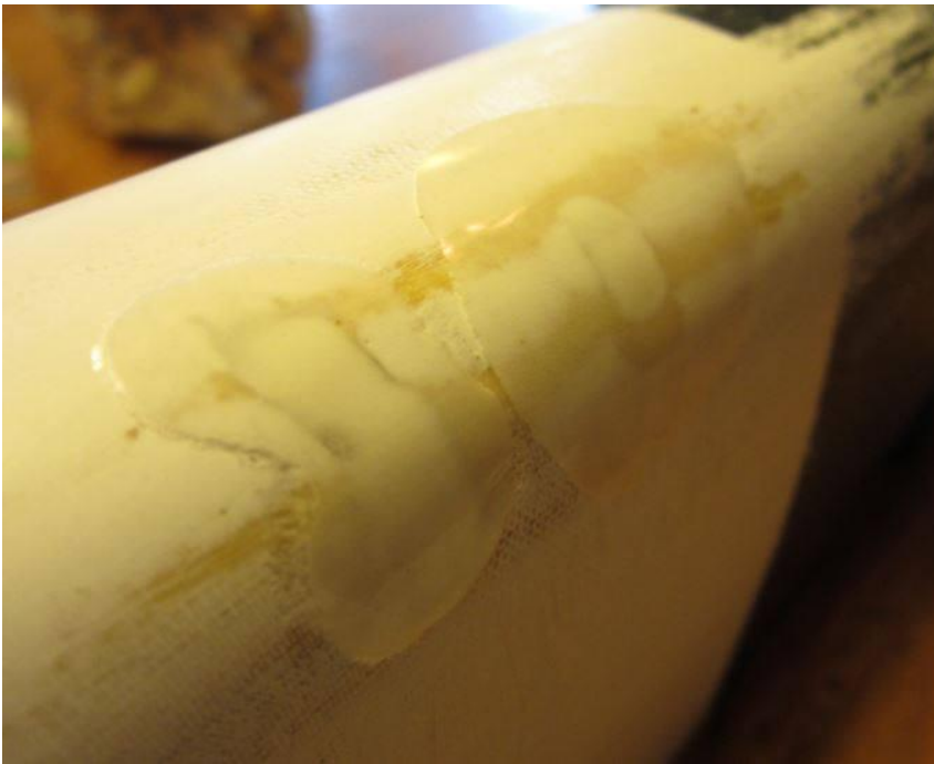
Here, the second application of filler cured with plastic removed.
