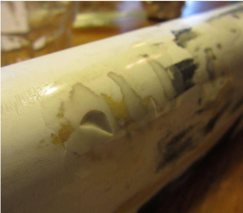
Here's the first application of cured filler repair.
